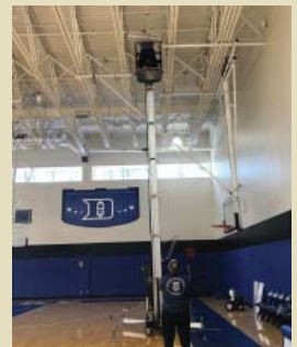
Justin Rook and Tommy Huff use a lift to change the lights.
