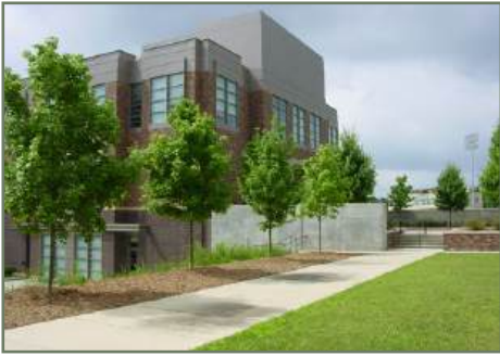
Yoh Football Entry Plaza and Courtyard
