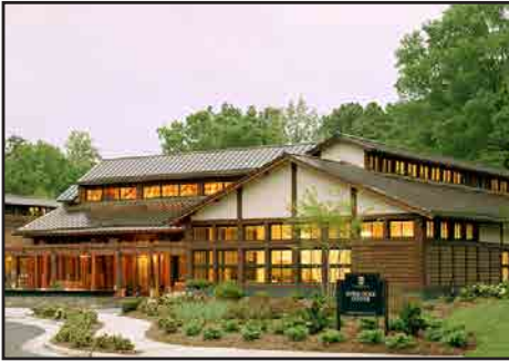
Doris Duke Center 2001 Atkin Olshin Lawson-Bell & Associates Duke Gardens Visitor Center 10,645 sf
