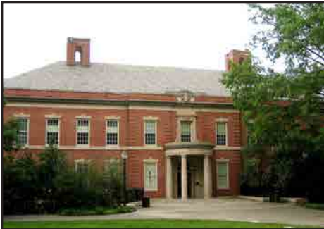
Hudson Hall 1948 Office of Horace Trumbauer Pratt School of Engineering 87,022 sf
