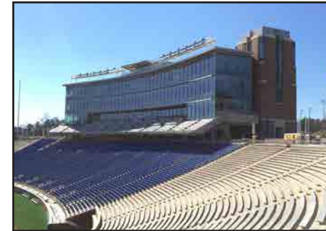
Blue Devil Tower 2016 The Beck Group Football Operations 95,000 sf LEED Silver
