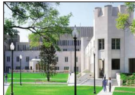
Original Hospital South Duke Clinic Renovation 1999 Cooper Robertson and Partners Medical Clinics 607,299 sf
