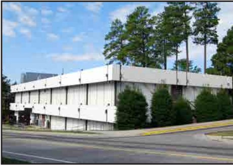
Research Park Buildings 1968-1970 John D. Latimer and Associates Research Labs and Offices 55,726 sf
