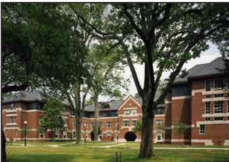
Blackwell Residence Hall 1994 Architectural Resources Cambridge Inc/ Little and Associates Architects Student Residence (194 Beds) 47,191 sf
