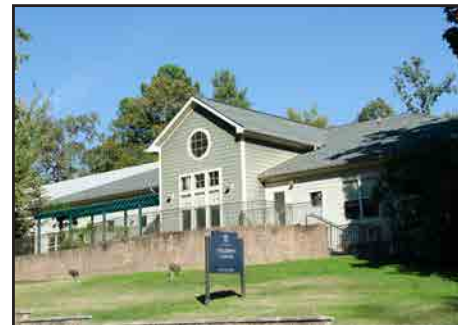
Children's Campus Expansion 2004 Winstead Wilkinson Architects Day Care 13,503 sf Originally built in 1995
