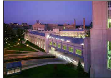
Duke Clinic Reception Building & Bridge 1999 Cooper Robertson and Partners Medical Clinics 102,930 sf
