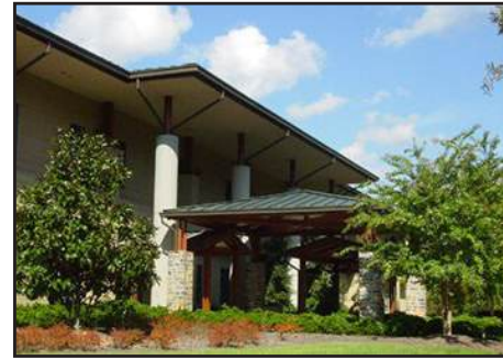
Wallace Clinic at the Center for Living 1991 Isley Architects Medical Clinics 15,453 sf
