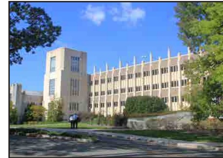
Parking Garage for Duke Clinic 1995 Cooper Robertson and Partners Parking Deck (1,794 spaces) 594,916 sf
