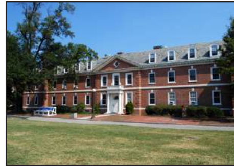
Wilson Residence Hall 1927 Office of Horace Trumbauer Student Residence (109 Beds) 47,712 sf
