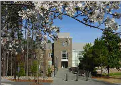
Law School Addition 2005 Dagit Saylor Architects Law School 28,200 sf LEED Certified
