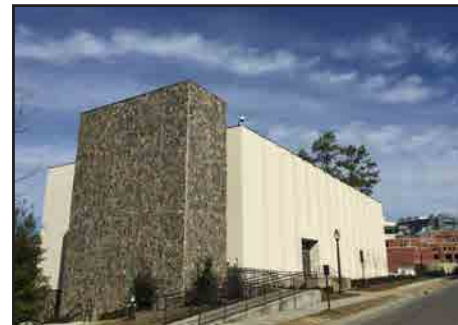
Telcom Building Renovation 2016 Brockwell Associates Office of Information Technology 26,680 sf
