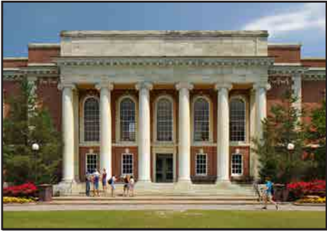
East Union Marketplace Renovation 2015 Clark Nexsen Dining Hall 44,196 sf
