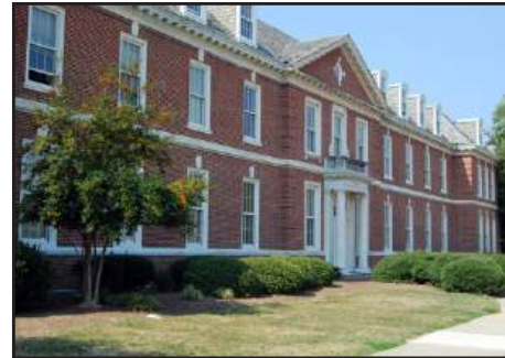
Carr Building 1927 Office of Horace Trumbauer Office and Classroom Space 53,781 sf
