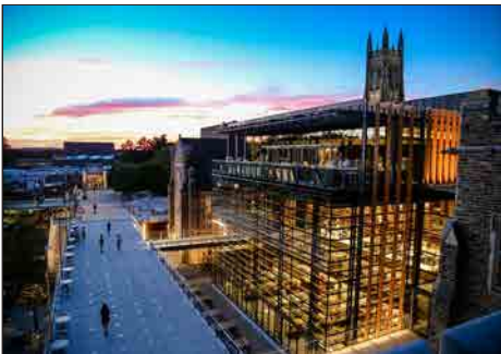
West Union 2016 Grimshaw Architects Student Union and Dining 124,770 sf LEED Silver
