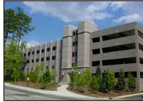
Bryan Center Parking Garage 2004 Walker Parking/ Cooper Robertson and Partners Parking Deck (545 spaces) 226,357 sf
