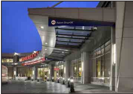
Emergency Department Expansion 2007 Perkins Eastman Hospital 56,770 sf
