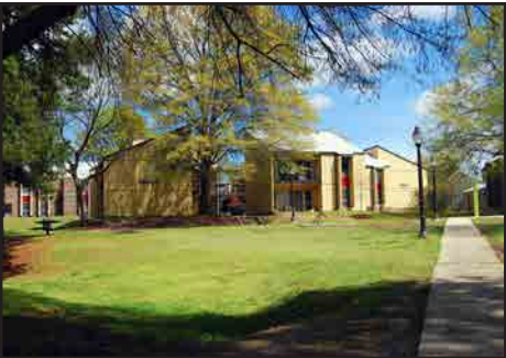
Central Campus Apartments Renovations 2010 J Davis Architects Student Residence (1050 Beds) 415,155 sf
