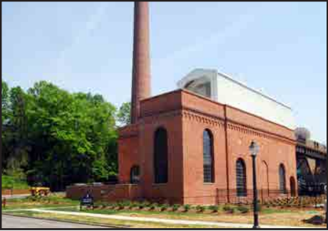
East Campus Steam Plant 2010 Smith Group JJR Steam Production 13,598 sf LEED Gold
